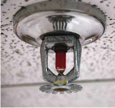
An example of a commercial fire sprinkler, (left), and a concealed residential sprinkler head (below).
