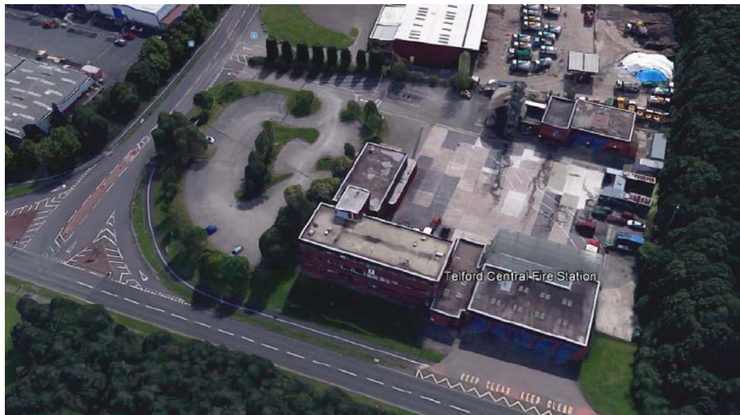
Fig 1. Aerial view of the site looking southwards
